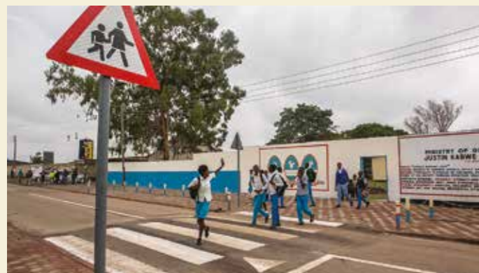
Vaccine implemented: after design changes, including speed humps, traffic speeds have been reduced to below 30km/h.
