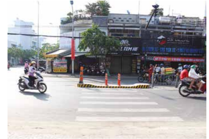
New refuge island installed after a SR4S assessment in Ho Chi Minh City, Vietnam.
